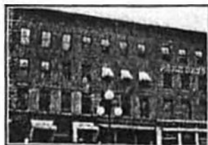
On the upper floor of this building, over the Park Drug Store, the Convocations of Burlington, Vt., College Photo by Allan
